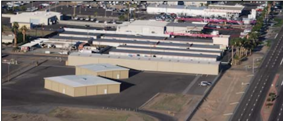
Figure 23 - Northwest GA Hangars
