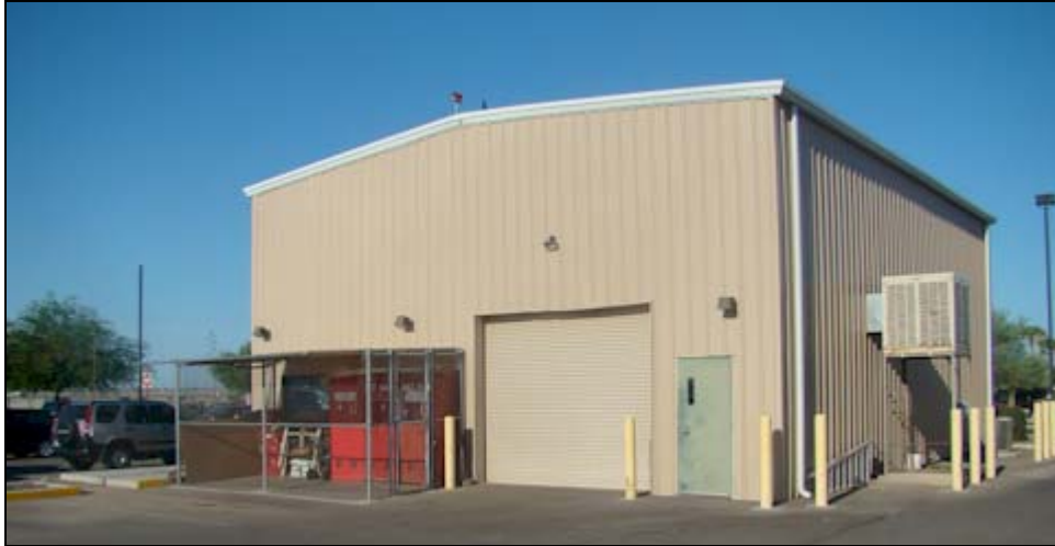
Figure 15 - Hertz Rental Car Service Facility
